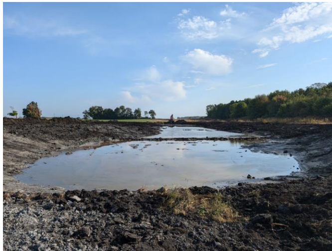
2-acre wetland in Muirkirk, under construction
