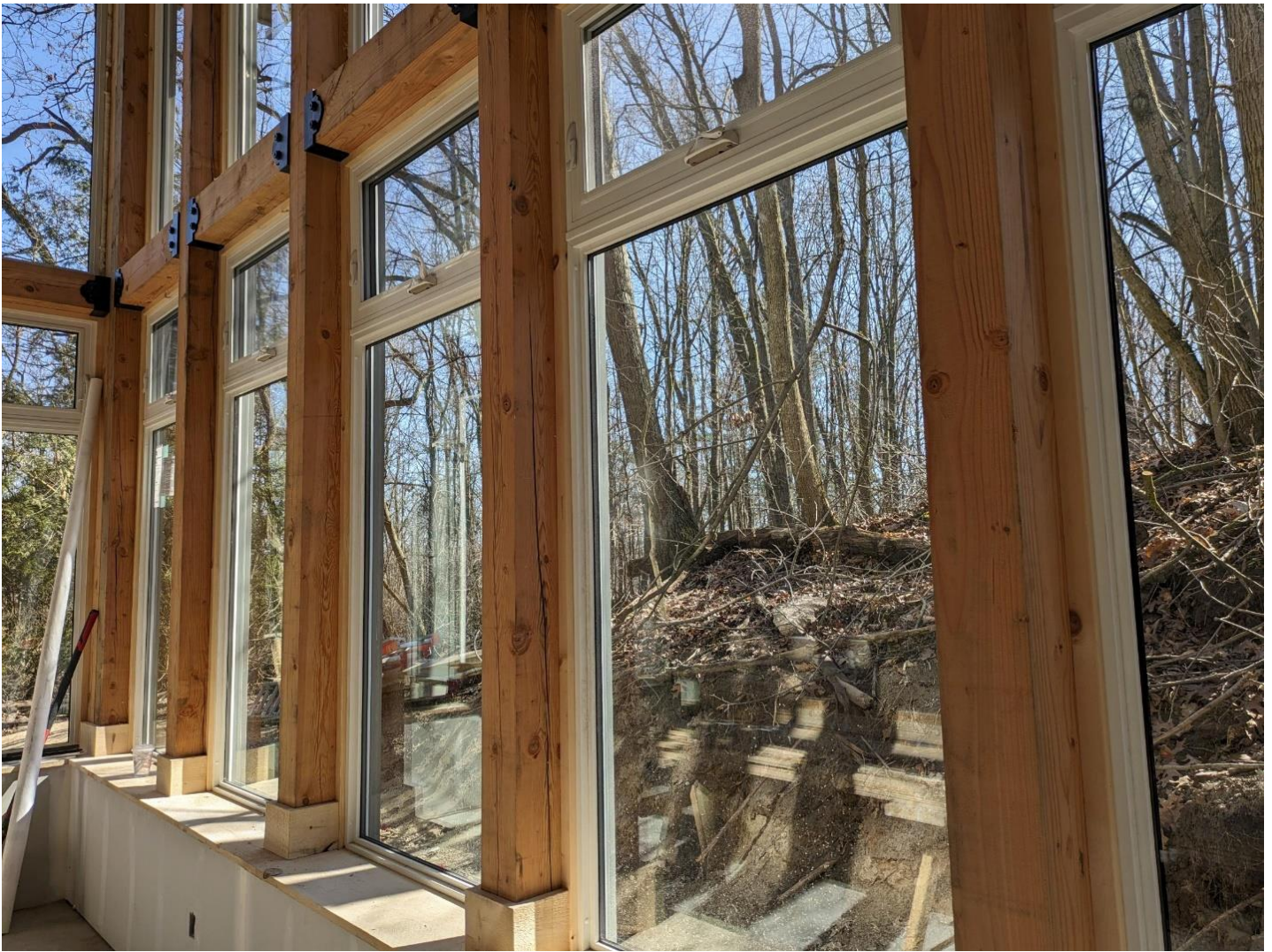
Longwoods RC Hall- Window and Beam Work
