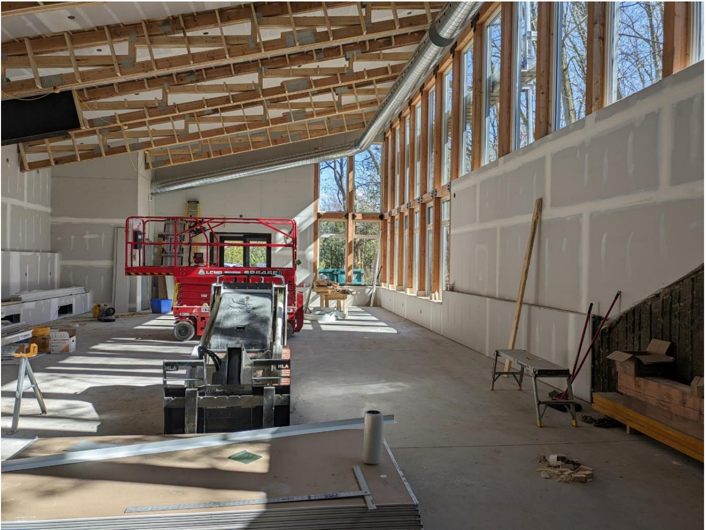
Longwoods RC Hall- Drywall Installation
