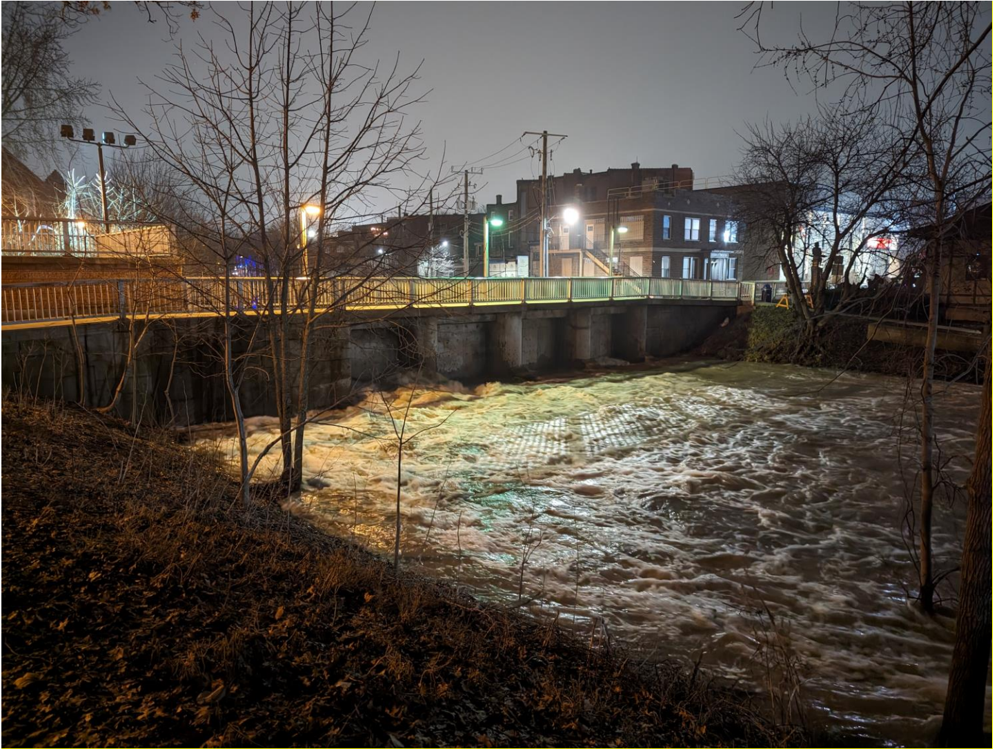
Photo: 6 th Street Dam and Pumping Station in operation on the evening of January 28 th .
