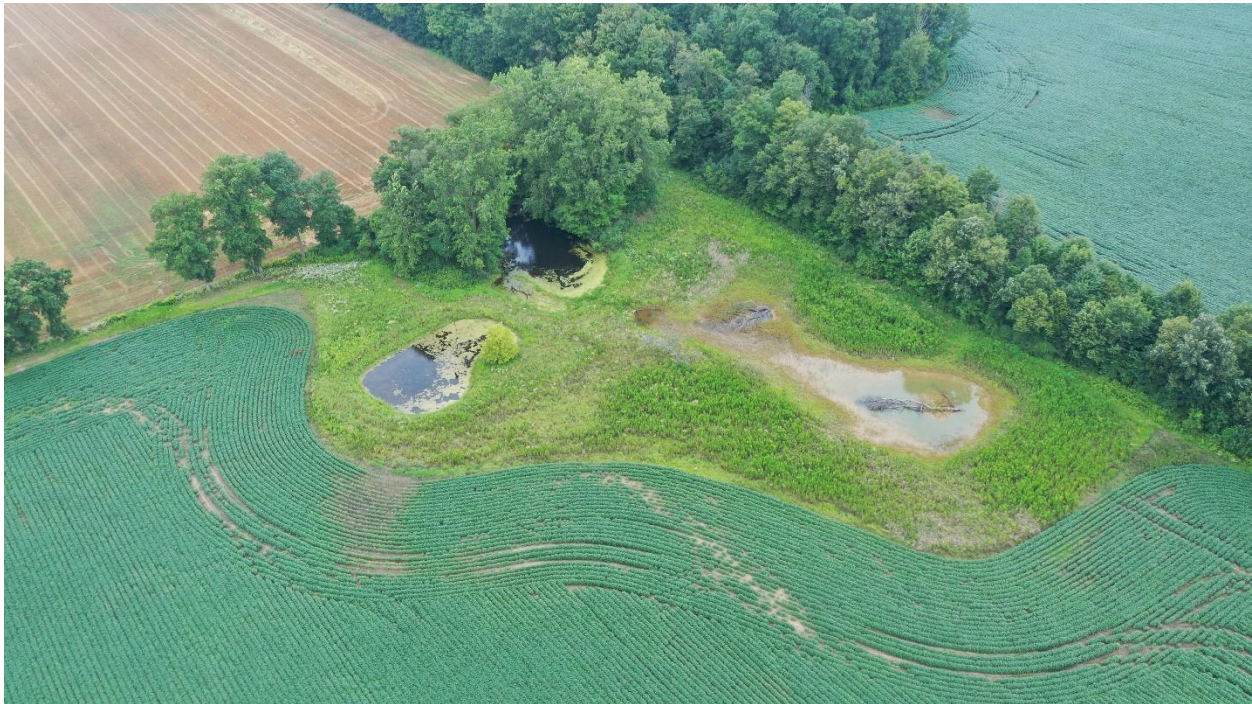
Figure 1 This project, completed 2022, already shows remarkable improvement. The wetland has already begun working, as it helps to hold and filter excess nutrients (visible algae) from entering the watershed.
