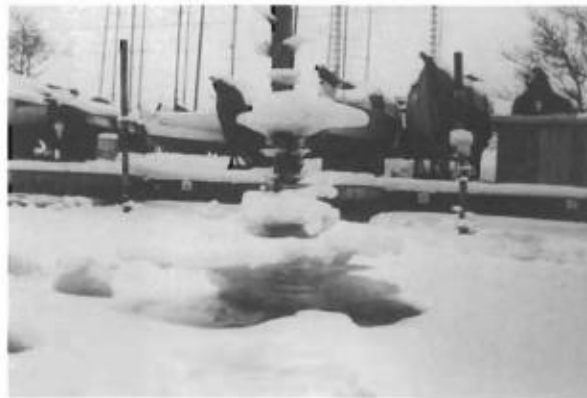
Figure 1. Pile damaged by vertical forces.
