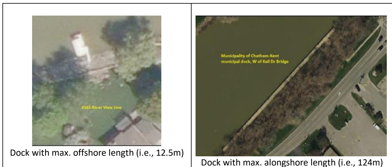
Figure 2.2: Selected Docks in the Lower Thames River (photos courtesy of LTVCA)
