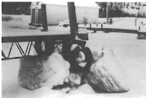
Figure 2. Rubble pile surrounding a pile with sufficient anchoring.
