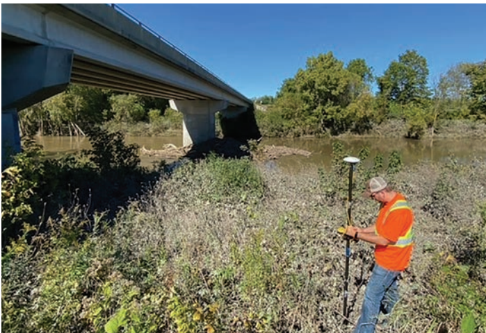
Jason Homewood – Water Resources and Regulations Technician surveyed flood markers along the Thames River following the September flood.
