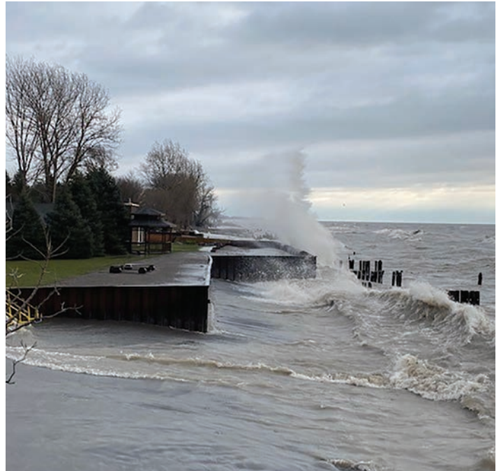
High lake levels pushed water up and over Lake Erie shoreline protection.
