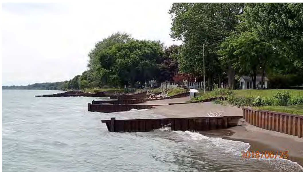
Figure 2.26 Steel Sheet Pile Groynes at Erie Beach
