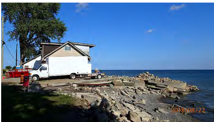
Figure 2.29 Dumped Concrete Rubble Shore Protection (2018.08.22)
