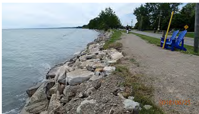
Figure 2.33 Armour Stone and Concrete Rubble in front of Dike, St. Anne's Church
