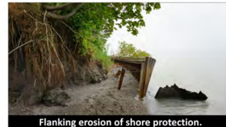
Flanking erosion of shore protection.
