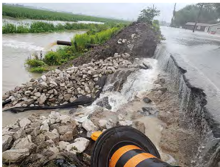
Figure 2.32 Erosion of Road Base, North Dike Slope and Flooding of Agricultural Fields, August 27, 2019 Storm
