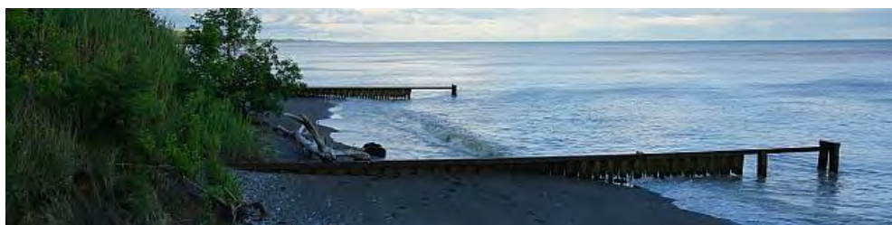
Figure 6.2 Steel Sheet Pile Groynes in Failure (top: sheet missing from the tip; bottom: vertical sheets corroded at the waterline)
