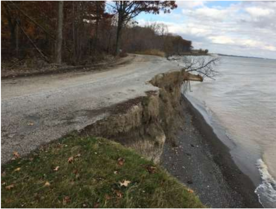
High water levels and storm-generated waves have greatly eroded the shoreline at southwestern Ontario parks, like Wheatley Provincial Park. (Jason Viau/CBC)
