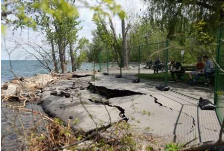
Pedestrians rest on a bench behind a fenced-off section of Hamilton's Waterfront Trail that collapsed due to high water levels and wave damage last year. (Dan Taekema/CBC)
