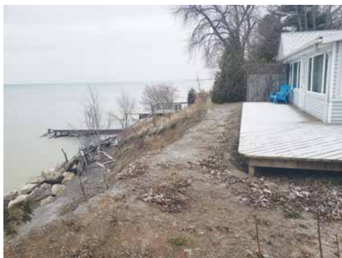
This is a view of a residential structure in close proximity to the top-of-bank of the Lake Erie bluff where the shoreline protection had recently failed.
