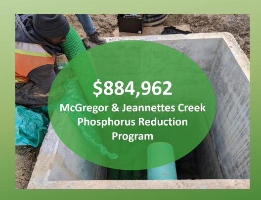
Installation of the Filtrexx Canada EnviroSoxx®, with NutriLoxx®, which is being tested at the TRPRC phosphorus filter tank pilot project site.
