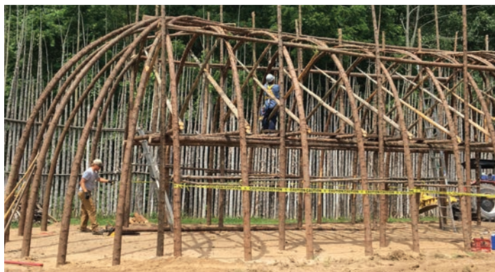
Two Heritage Build Labourers - Vance Stark and Rolland Pheasant assisted staff with preparing 34 central arches for the new longhouse.
