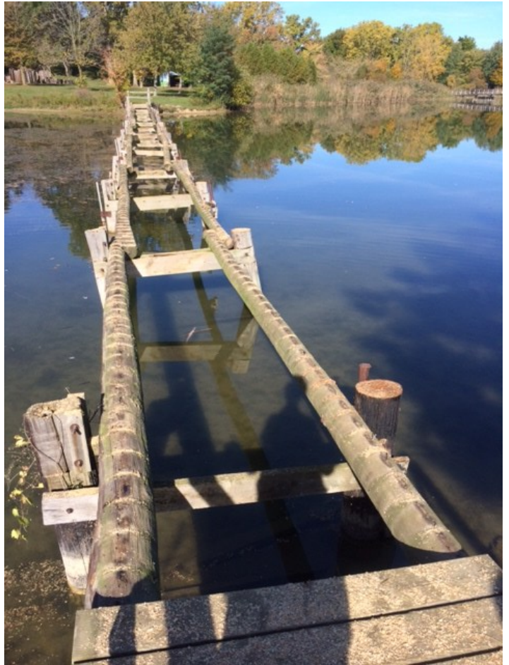
C.M. Wilson bridge in the process of being removed for earthen structure which is low maintenance and less liability.
