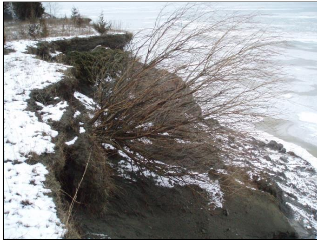
Shoreline Erosion- Failure of vegetation protection.
