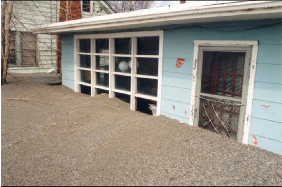
Structure located on an active dynamic beach (sand dune)-Erie Shore Drive.
