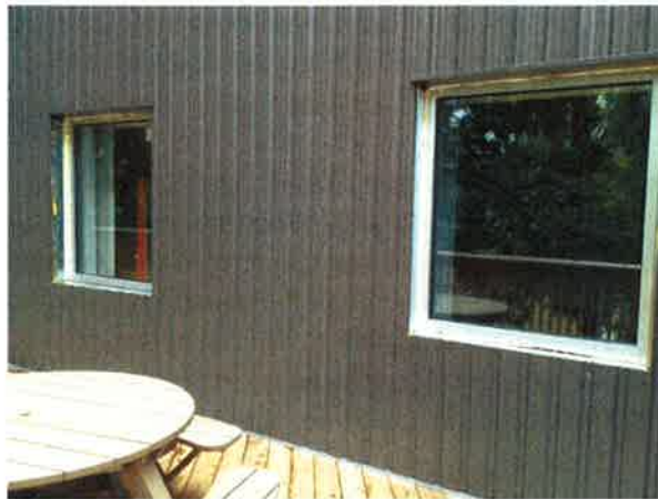
New windows being installed
