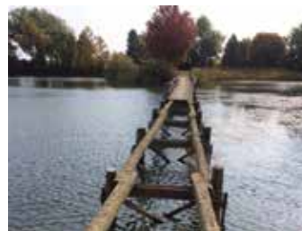
Dismantling C.M. Wilson boardwalk to create an earthen berm will result in a safe, naturalized shore.
