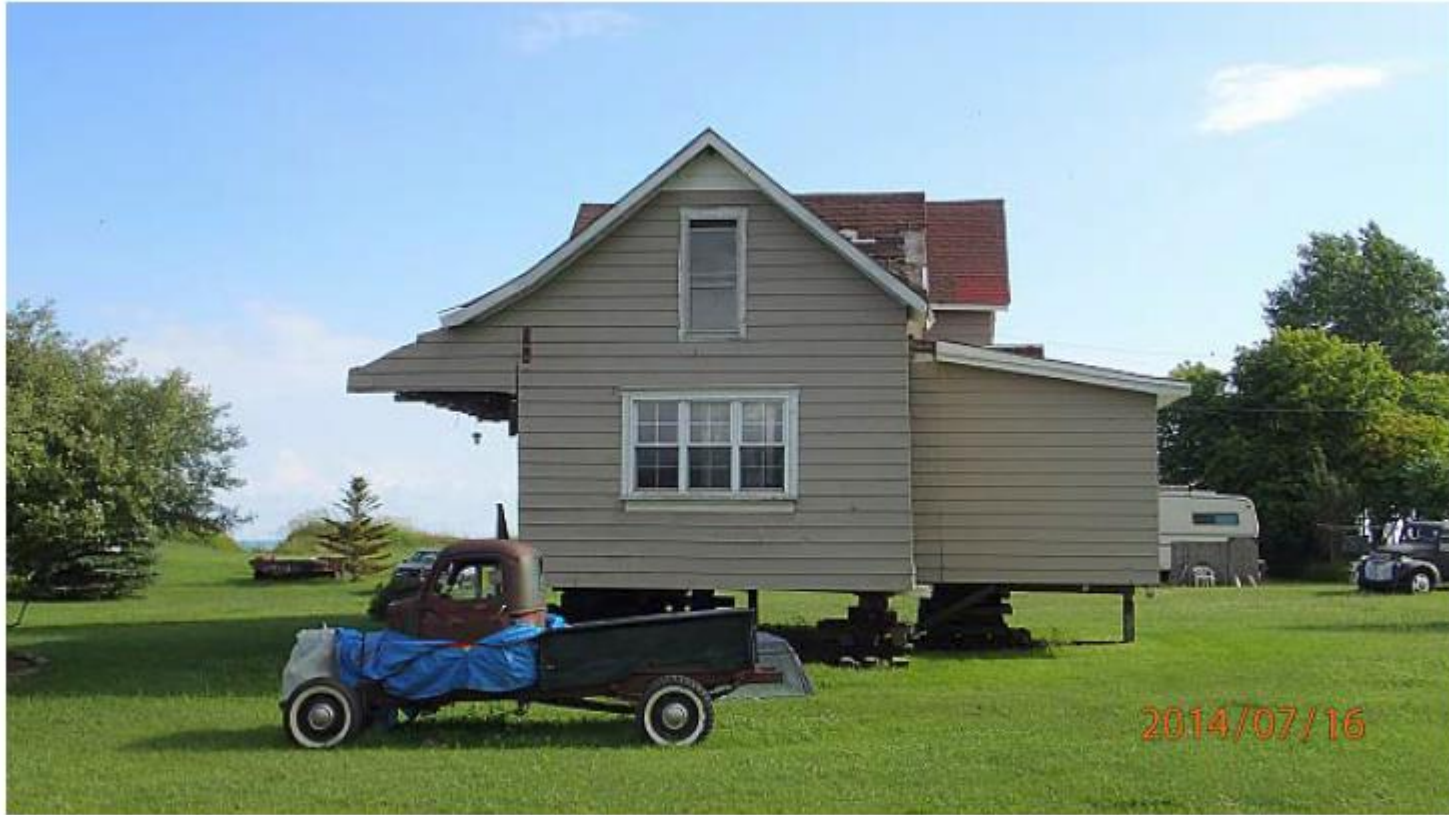
Home on Temporary Piles (assumed relocation due to bluff recession)
