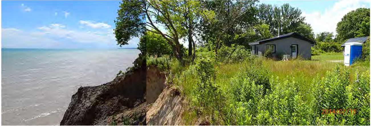
Figure 6.4 Building in Close Proximity to the Eroding Bluff Crest
