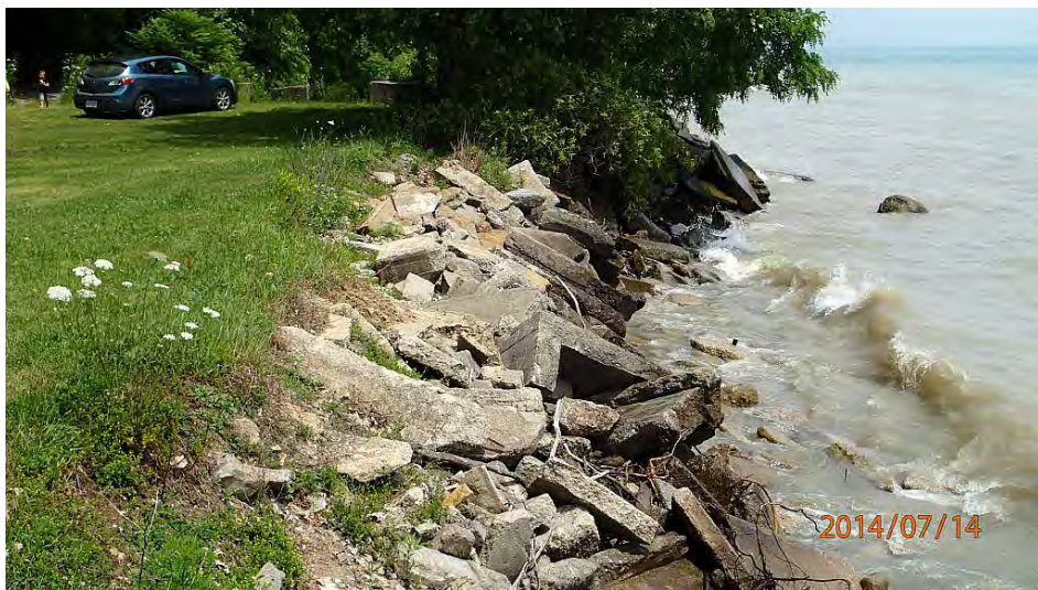
Figure 4.13 Ad Hoc Concrete Rubble Protection in Port Glasgow
