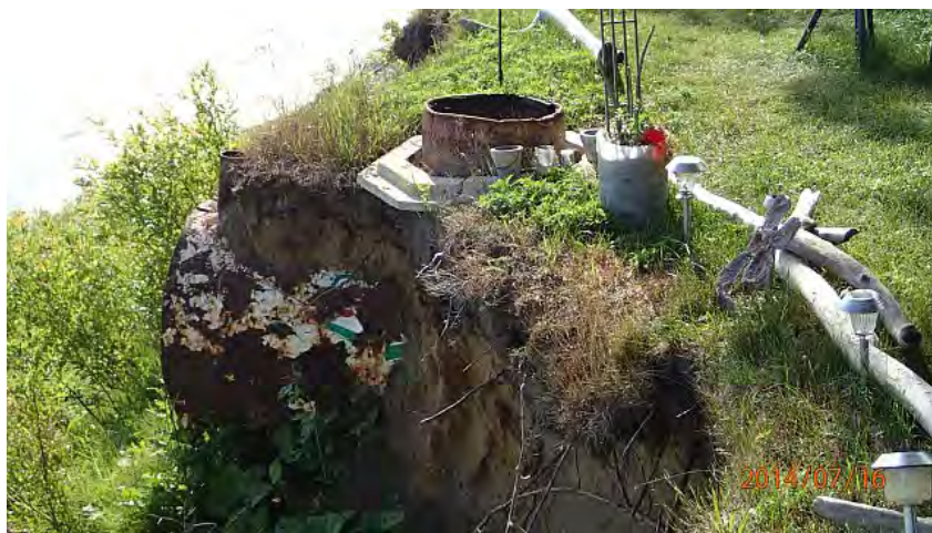
Figure C.4 Old Fuel Tank Exposed in Eroding Bluff Crest
