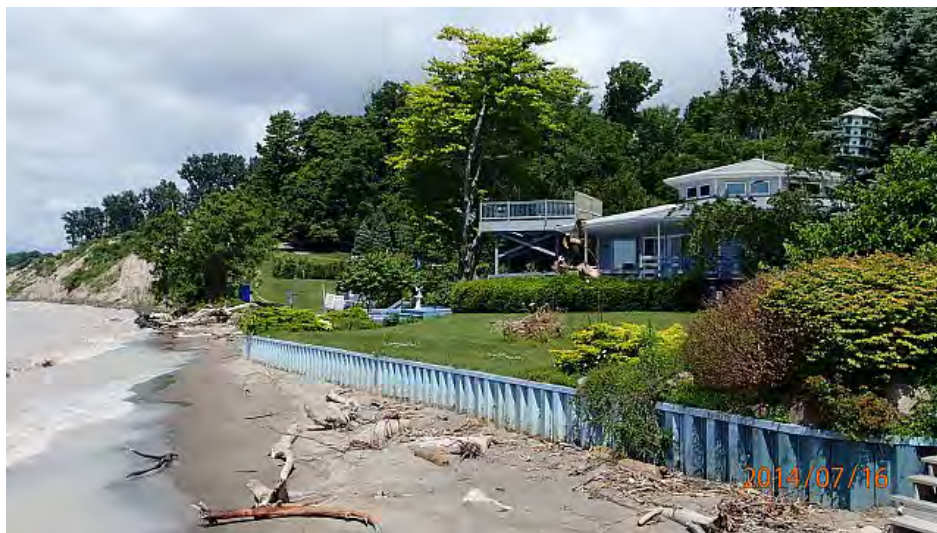
Figure 7.5 Steel Sheet Pile Wall Protecting Residential Development in CCCA Reach 1
