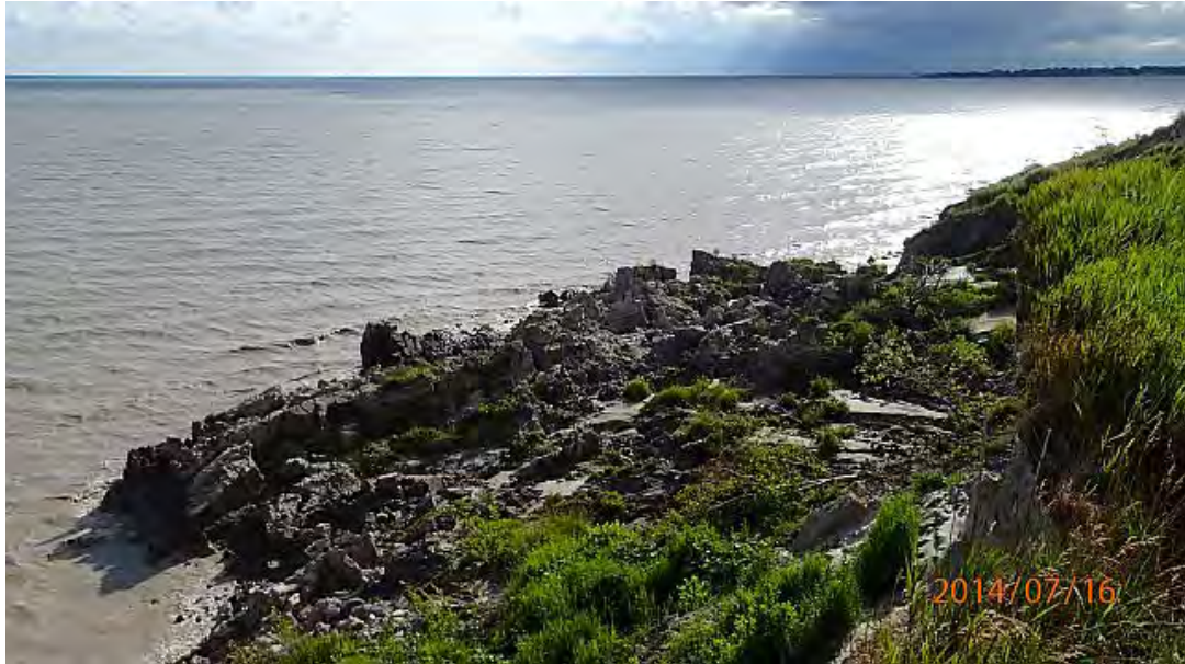
Figure 2.9 Debris from a Massive Bluff Failure East of Port Burwell
