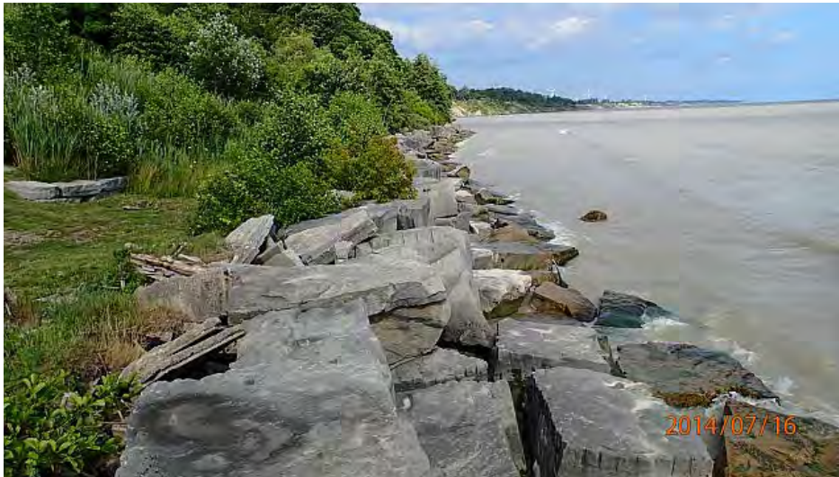
Figure 4.11 Armour Stone Revetment East of the Navigation Channel, Port Burwell
