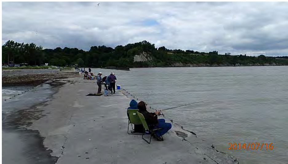
Figure 7.8 Western Jetty in Port Bruce
