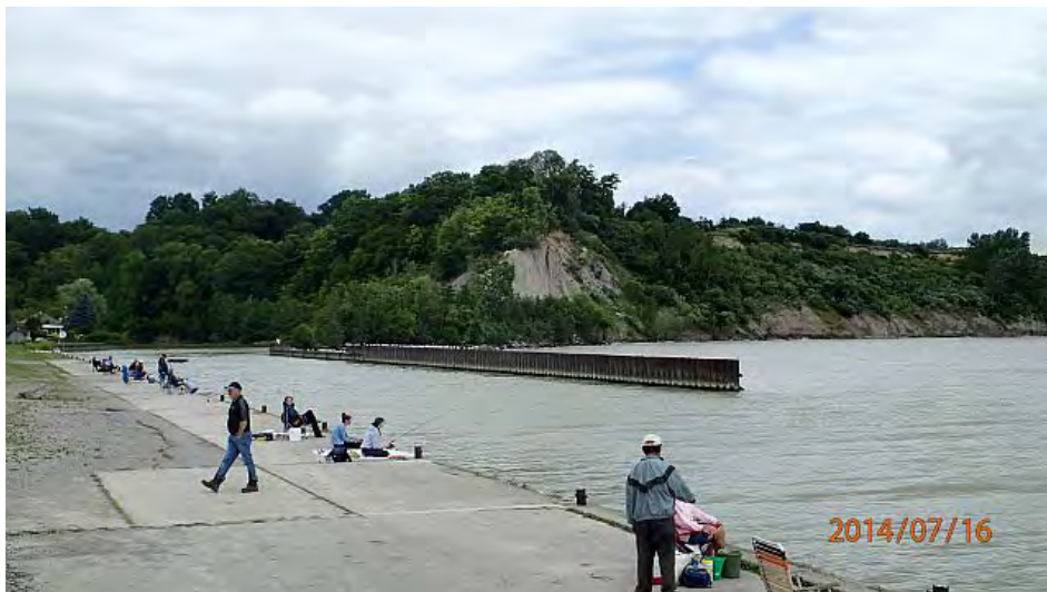
Figure 4.7 View of Port Bruce Jetties and Navigation Channel Looking Upstream
