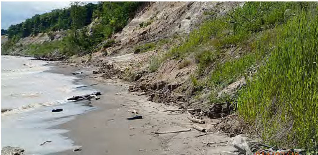
Figure 2.8 Toe Erosion due to Wave Attack (east of Port Bruce)
