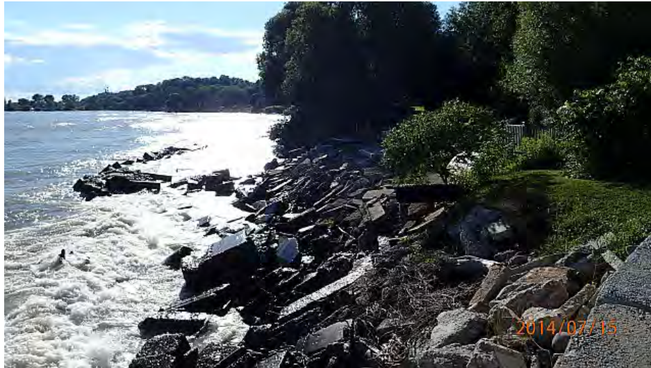
Figure 6.10 Existing Dumped Concrete Rubble in KCCA Reach 4
