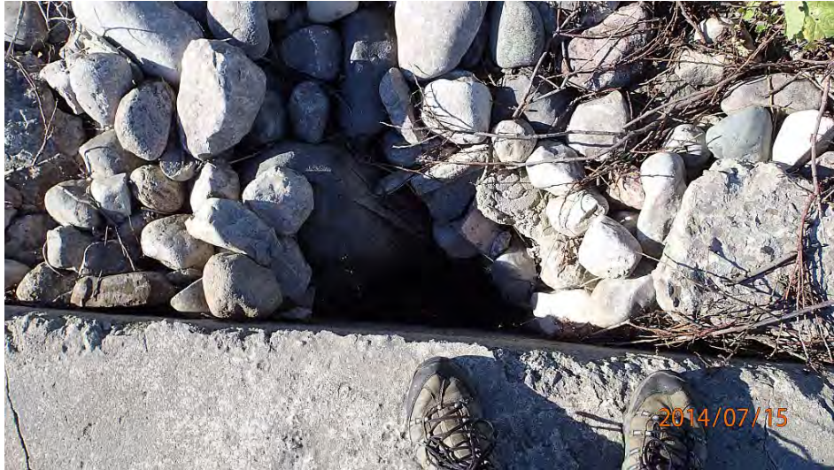
Figure 4.12 Cavity Behind a Concrete Block Wall in Port Stanley
