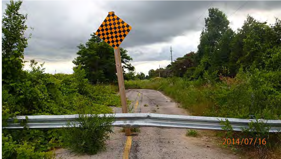
Figure 8.5 Section of Lake Shore Line Closed Due to the Erosion Hazard
