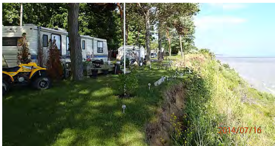
Figure C.2 Trailers Located in Close Proximity to the Bluff Crest
