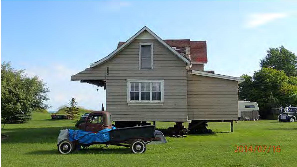
Figure 4.2 Home on Temporary Piles (assumed relocation due to bluff recession)
