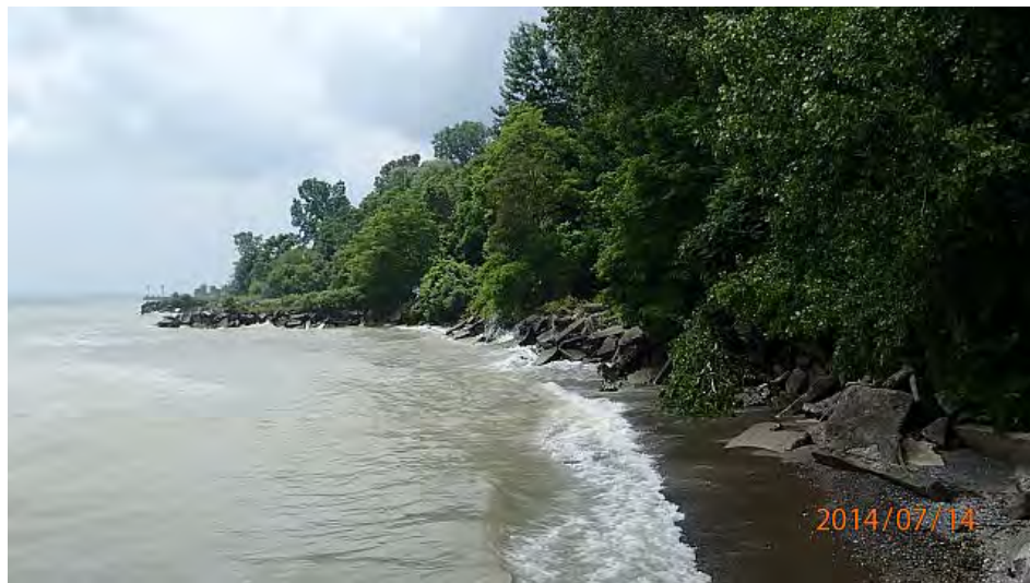
Figure 5.5 Concrete Rubble Shoreline Protection East of Navigation Channel, Port Glasgow
