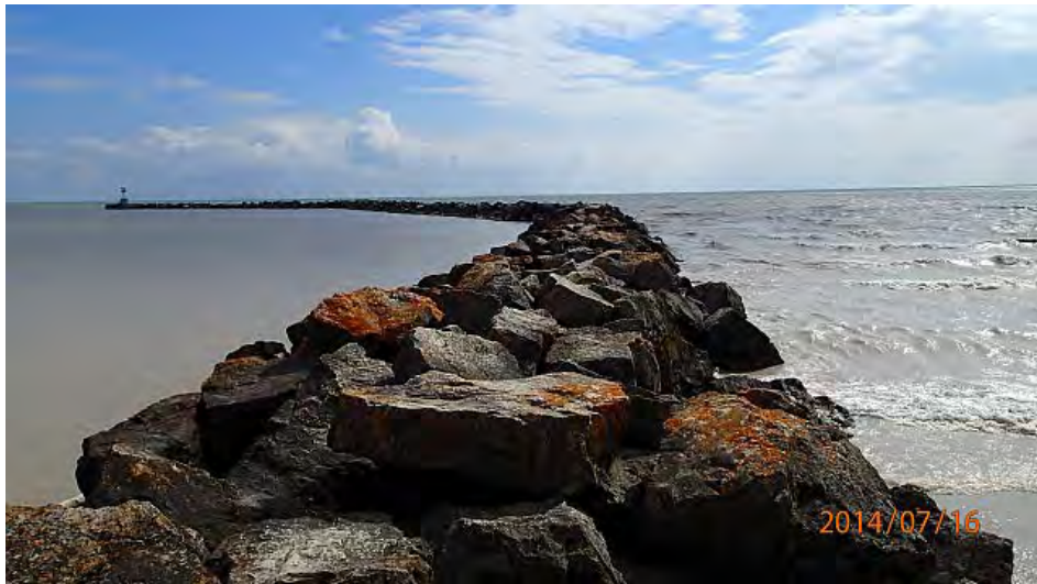
Figure 8.7 Armour Stone Jetty Extension (west jetty) at Port Burwell
