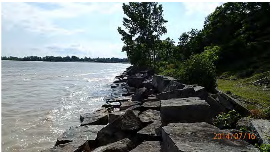
Figure 8.10 Armour Stone Revetment at the Foot of Pitt Street
