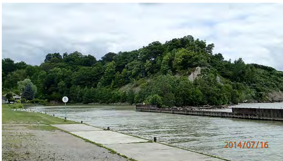
Figure 7.9 Eastern Jetty at Port Bruce and Protection at the Toe of Bluff
