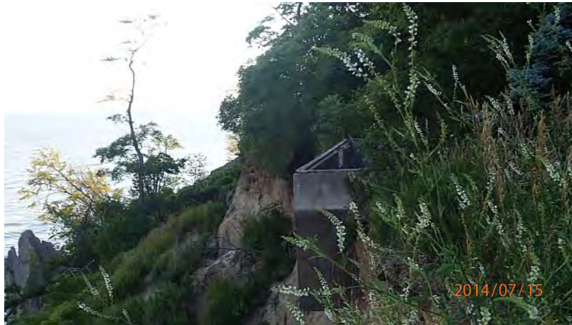
Figure C.3 Concrete Foundation from Abandoned House Exposed in Bluff Crest
