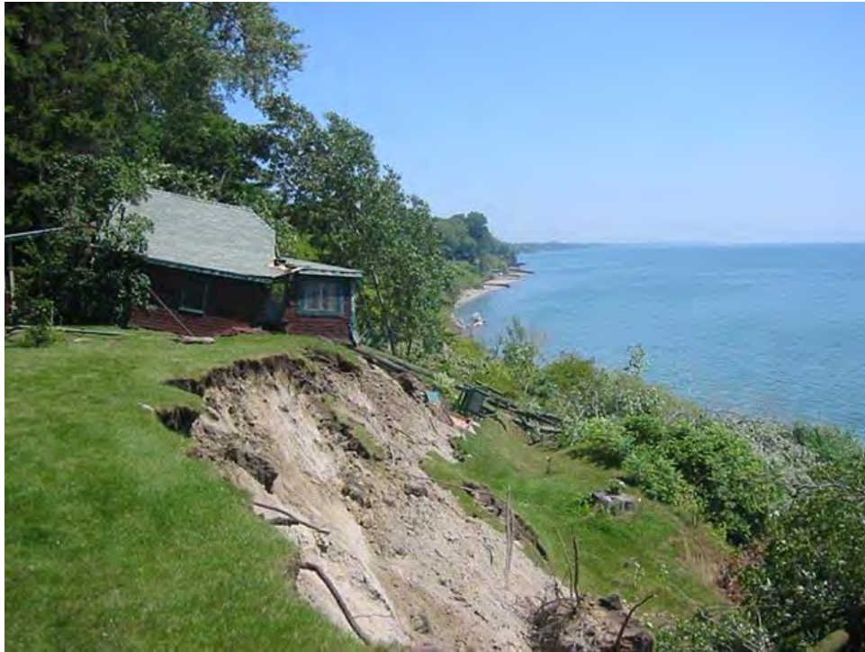
Figure 3.1 Home Destroyed by Bluff Failure in the LTVCA (photo courtesy of the LTVCA)
