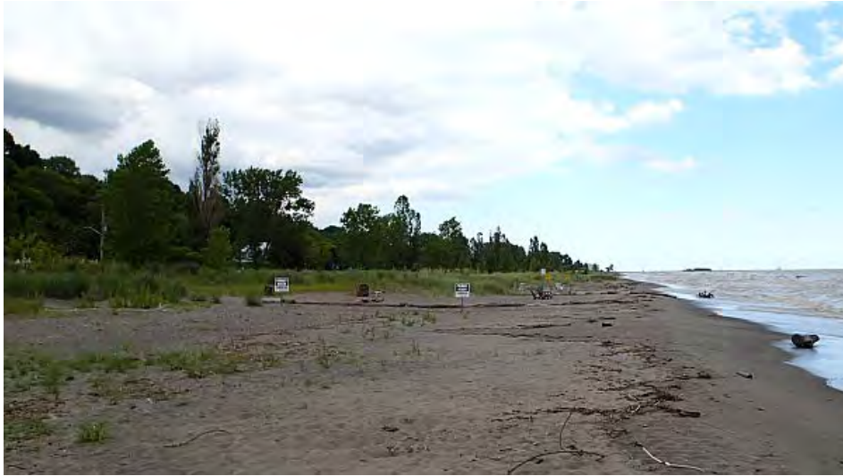
Figure 6.7 Beach and Dune Conditions in the Western Half of KCCA Reach 2
