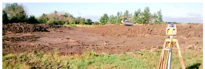
Wetland Construction on Lagoon Rd in Chatham-Kent on August 27 th .
