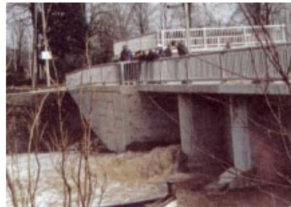
Dam and pumping station Indian/McGregor Creek Flood Control Project
