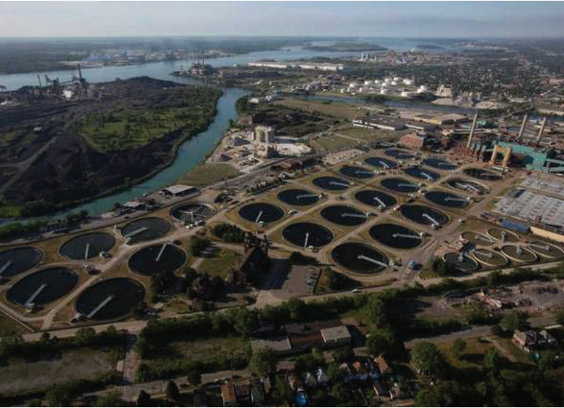
Detroit Wastewater Treatment Plant — In 2012, the plant was responsible for 7.8 billion gallons of untreated or partially treated sewage into the Detroit River.
